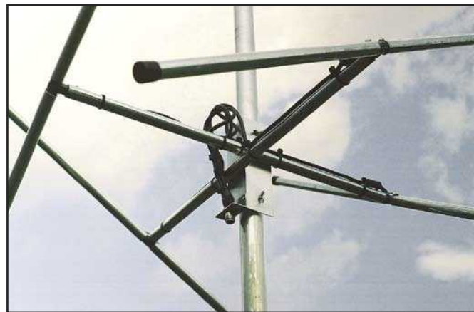
Figure 3 — View of cross booms mounted to mast.
