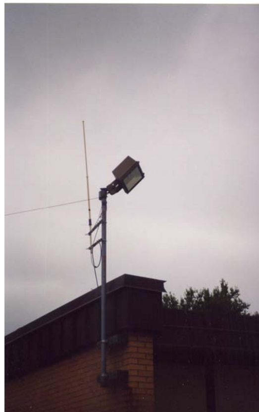
The antennas on Burbank School
