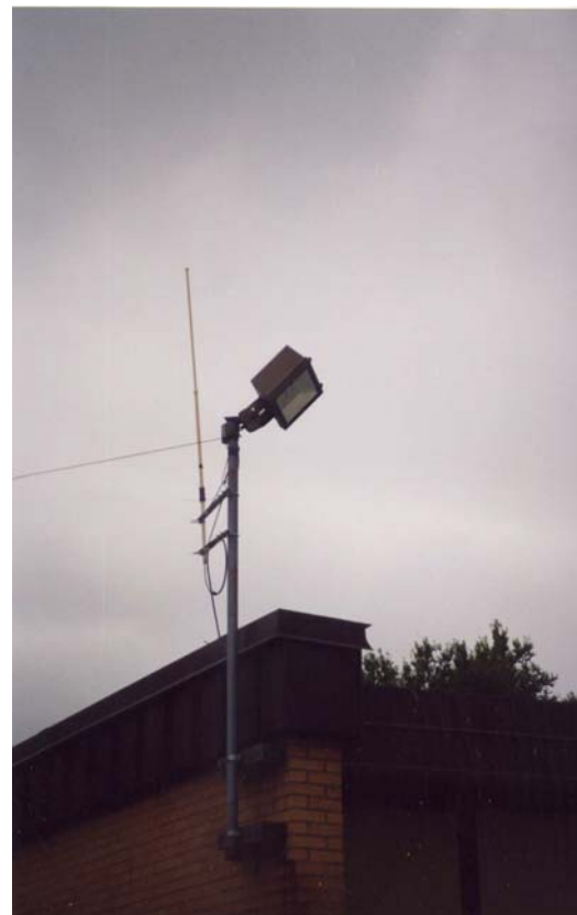
The antennas on Burbank School
